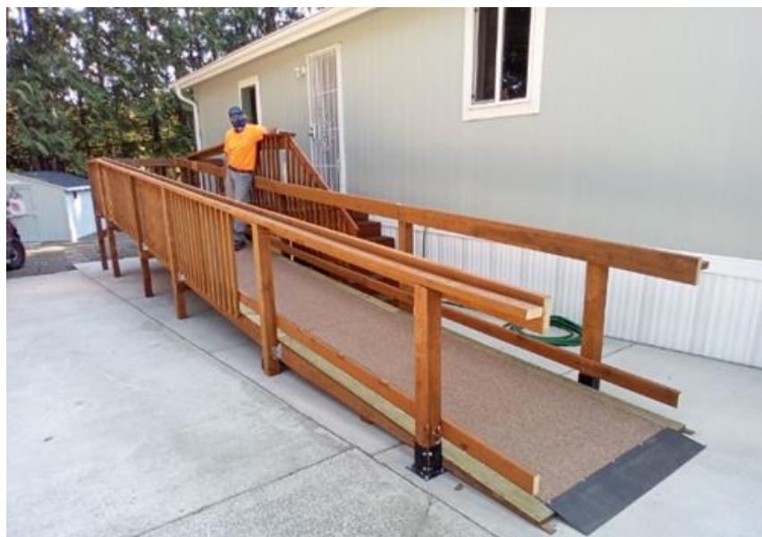
Nearly completed ramp
