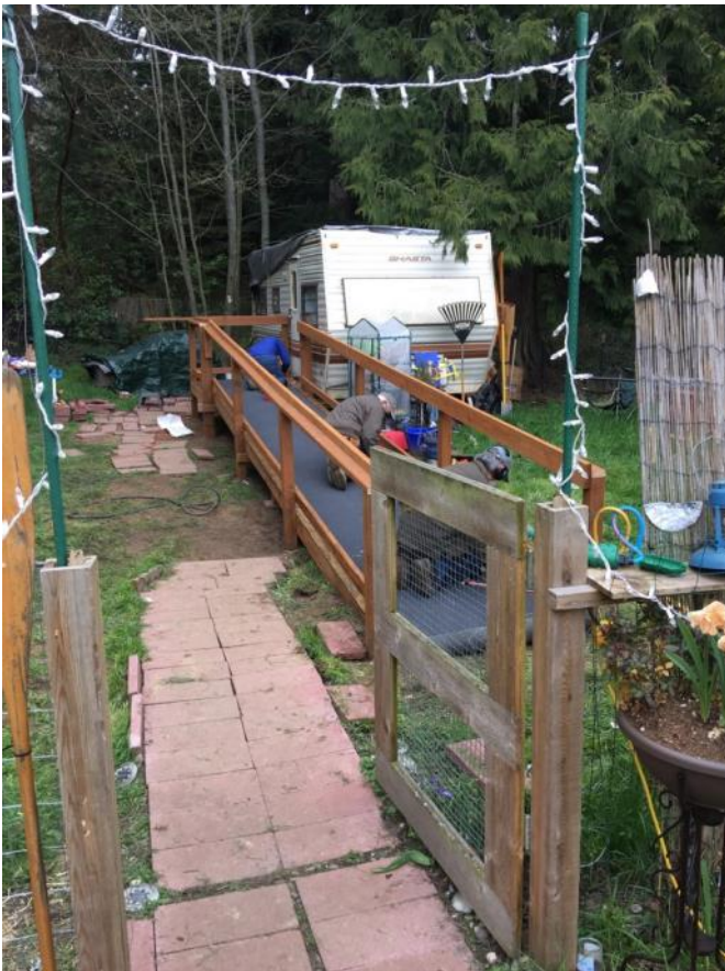
The crew installing a non-skid surface on the ramp.
