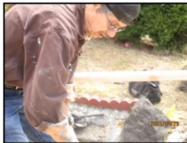
Tim Ruddy working on the supports.
