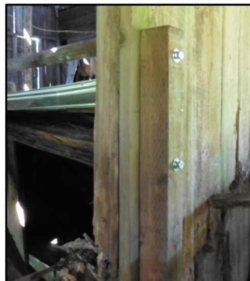
New posts spliced in with 1/2" rods
