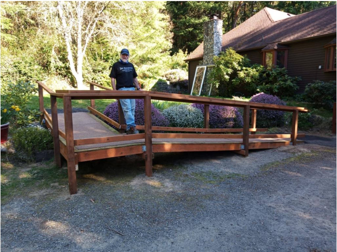
Michael Crovitz with the finished ramp (John White took the picture)
