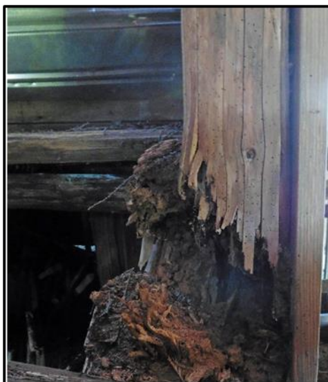
One of the rotted posts
