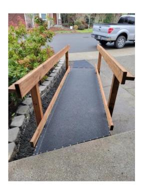
Left - Bluebills builders fund provided the materials for this low income client in Port Orchard. A 12' ramp was installed and steps with a lower rise were built.
