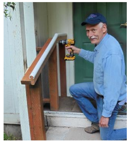
Marty Dasler installing a railing in Poulsbo
