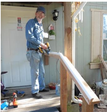
Mark Washeleski installing a railing in Port Orchard
