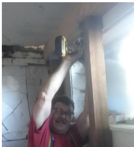
Greg DeVault – emergency temporary repairs in Bremerton
