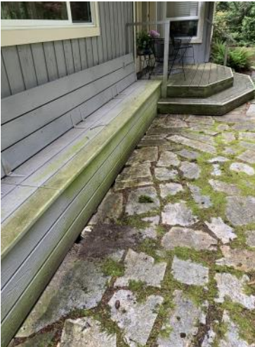
Bench to be removed to make room for the new ramp.
