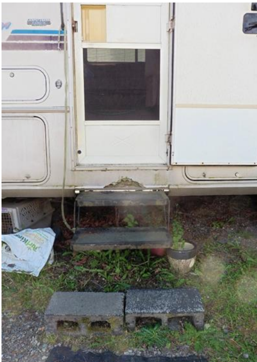
Dangerous stair steps at the Bremerton site
