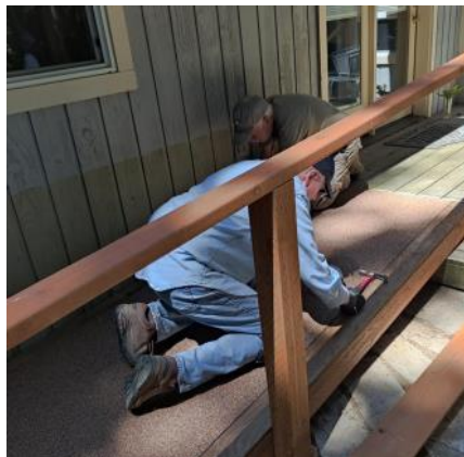
Jon and Mark put the finishing touches on the new ramp.
