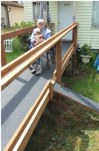
The ramp cut completely across the front yard
