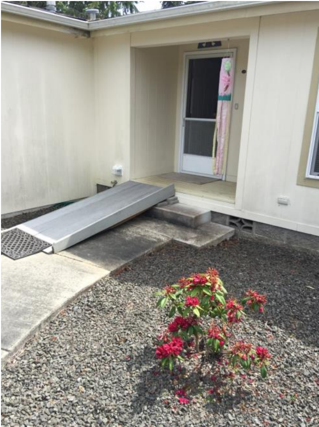
The existing ramp was not really adequate for the task.
