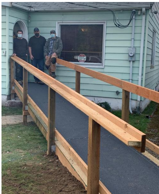
Greg DeVault, John White, and Bob Keever with the completed ramp.
