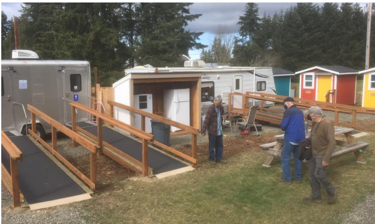
The three completed ramps. Two for the lavatory trailer and one for the kitchen trailer. Bluebills Todd Knoblock, John Fillers and Mark Cattabriga. Dan Nieuwsma took the photo.
