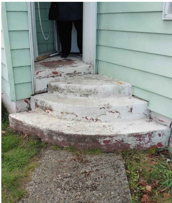
Dangerous concrete steps had no railing.
