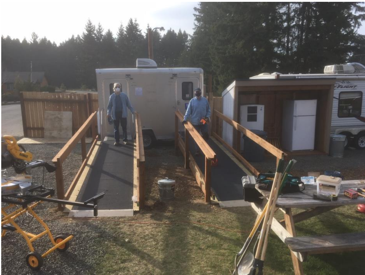
Todd Knoblock and John Fillers conducting structural integrity testing on the lavatory/shower facility ramps.
